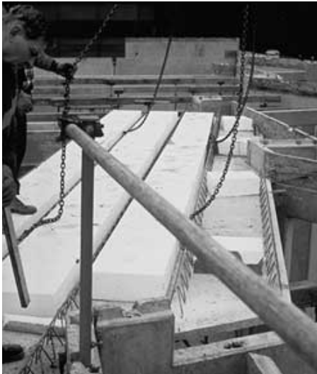
Figure 13: panels connecting to precast walls
