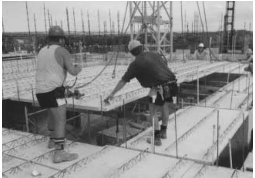
Figure 1: Placing a HumeSlab™ panel
