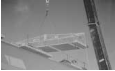
Figure 36: Cantilever portion of bridge deck is unpropped during construction
