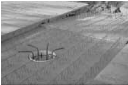
Figure 4: Column penetration in HumeSlab™ panel
