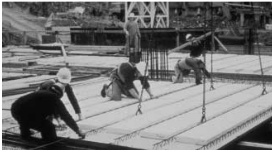
Figure 12: Slab and band beam system
