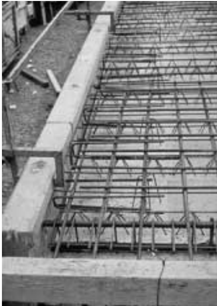
Figure 18: HumeSlab connecting to precast walls
