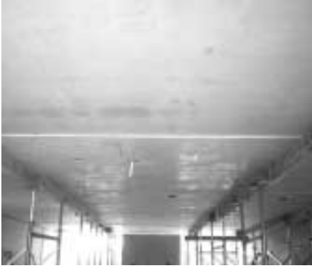
Figure 29: Unpainted soffit finish showing shadow joint
