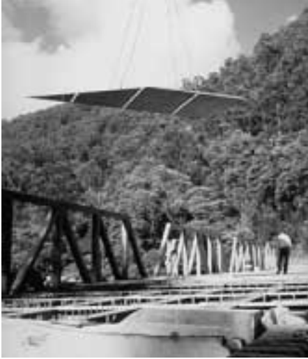
Figure 34: Thomson River Bridge - Victoria
