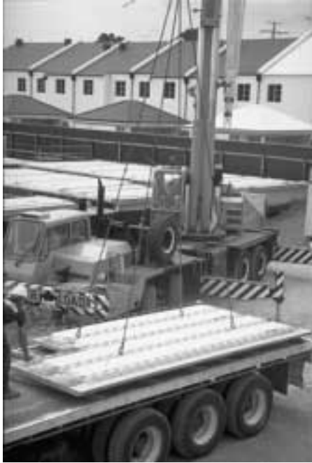
Figure 25: Site lifting - typical 4-point lift
