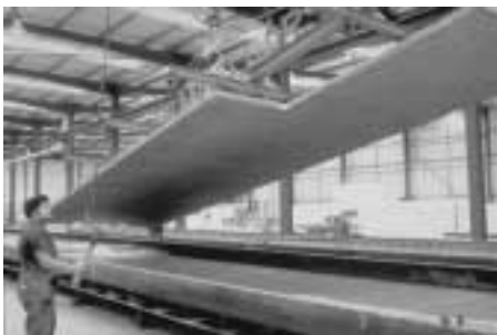
Figure 23: Lifting of HumeSlab panels from casting table
