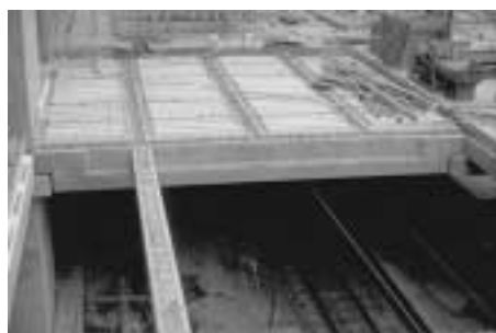
Figure 15: Unpropped HumeSlab™ panels on precast beams
