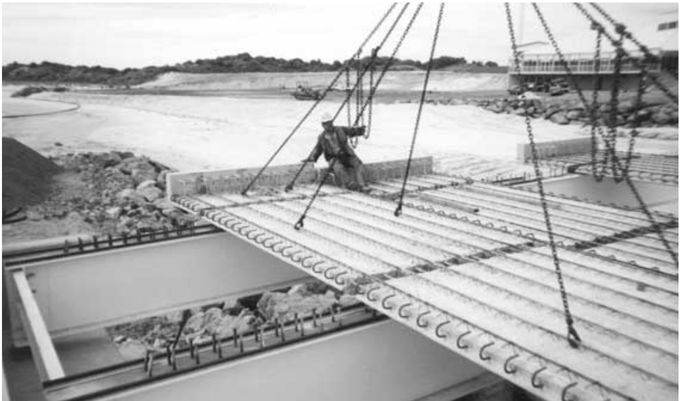
Figure 37: Placing bridge deck panels
