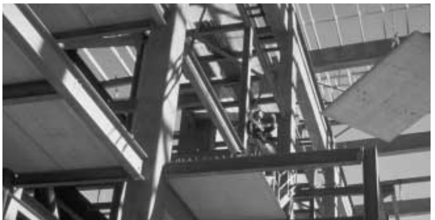
Figure 6: HumeSlab™ panels placed on steel frame structures
