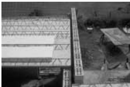
Figure 5: HumeSlab™ on load bearing block walls
